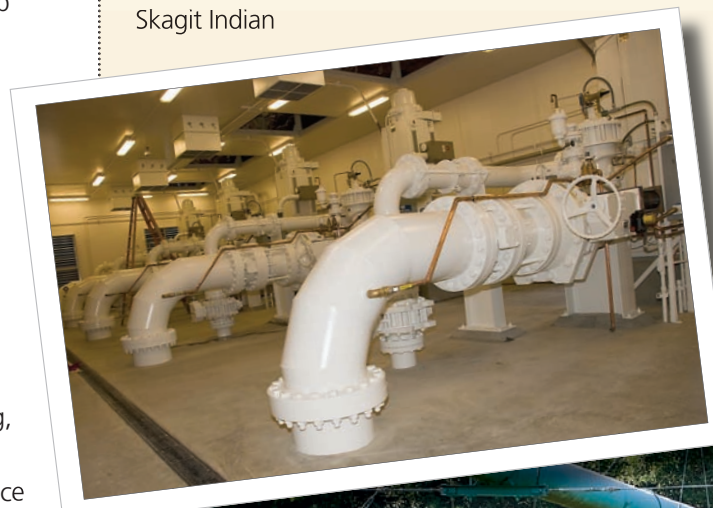
(Left) Five 900-horsepower engines will be able to deliver 36 million gallons of water per day to Judy Reservoir.
