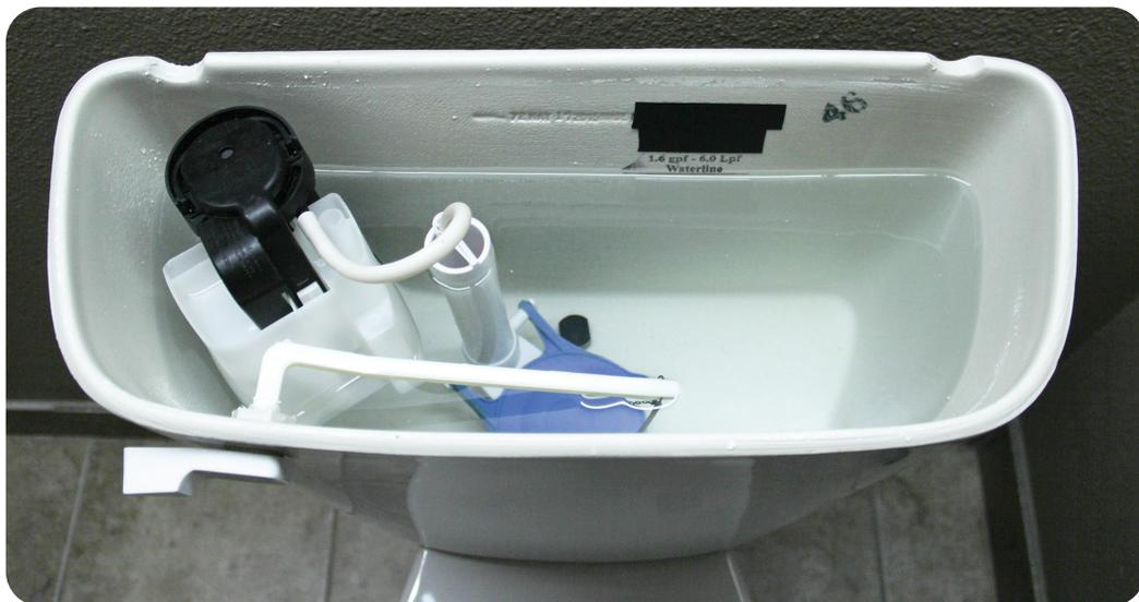
*Toilet flappers are the leading cause of leaking or running toilets — they provide the seal for the flush valve and control the volume of water released to the bowl.*
