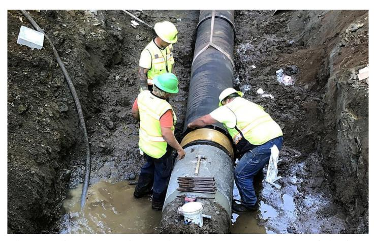
In this June 2019 photo, repairs are made to a 24-inch concrete water transmission pipeline near Morford Road east of Clear Lake.
