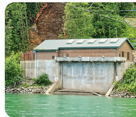
Skagit River Diversion Pump Station
