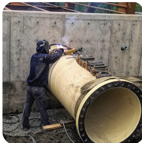
▲ A welder works on the pipeline section that crosses the Nookachamps Creek's East Fork. The PUD constructed a 200-foot single-span pedestrian bridge to support the pipeline over the creek. The bridge will be available for future use as part of Skagit County Parks & Recreation's planned Centennial Trail extension.
