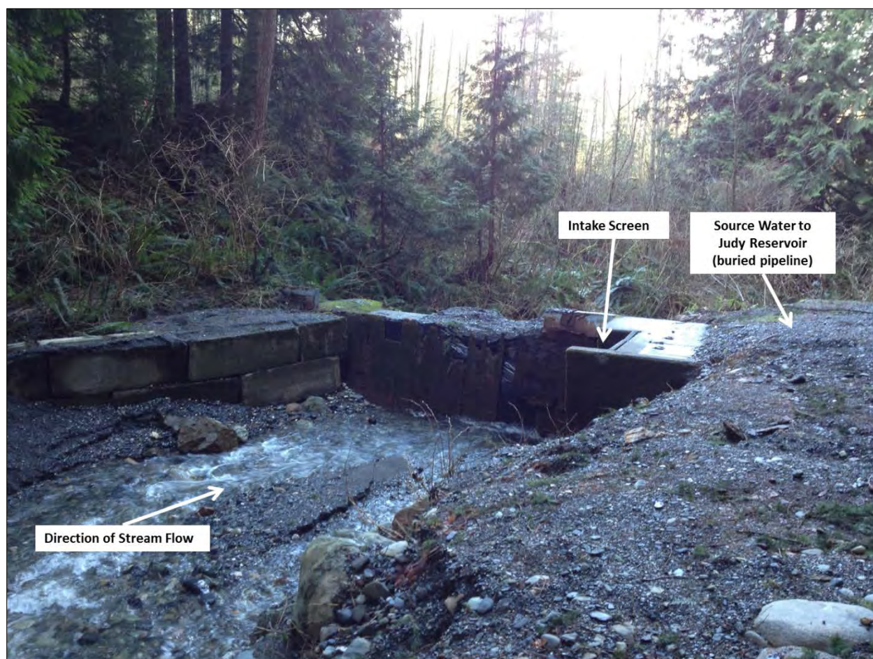
Figure 2-11. Turner Creek Diversion
