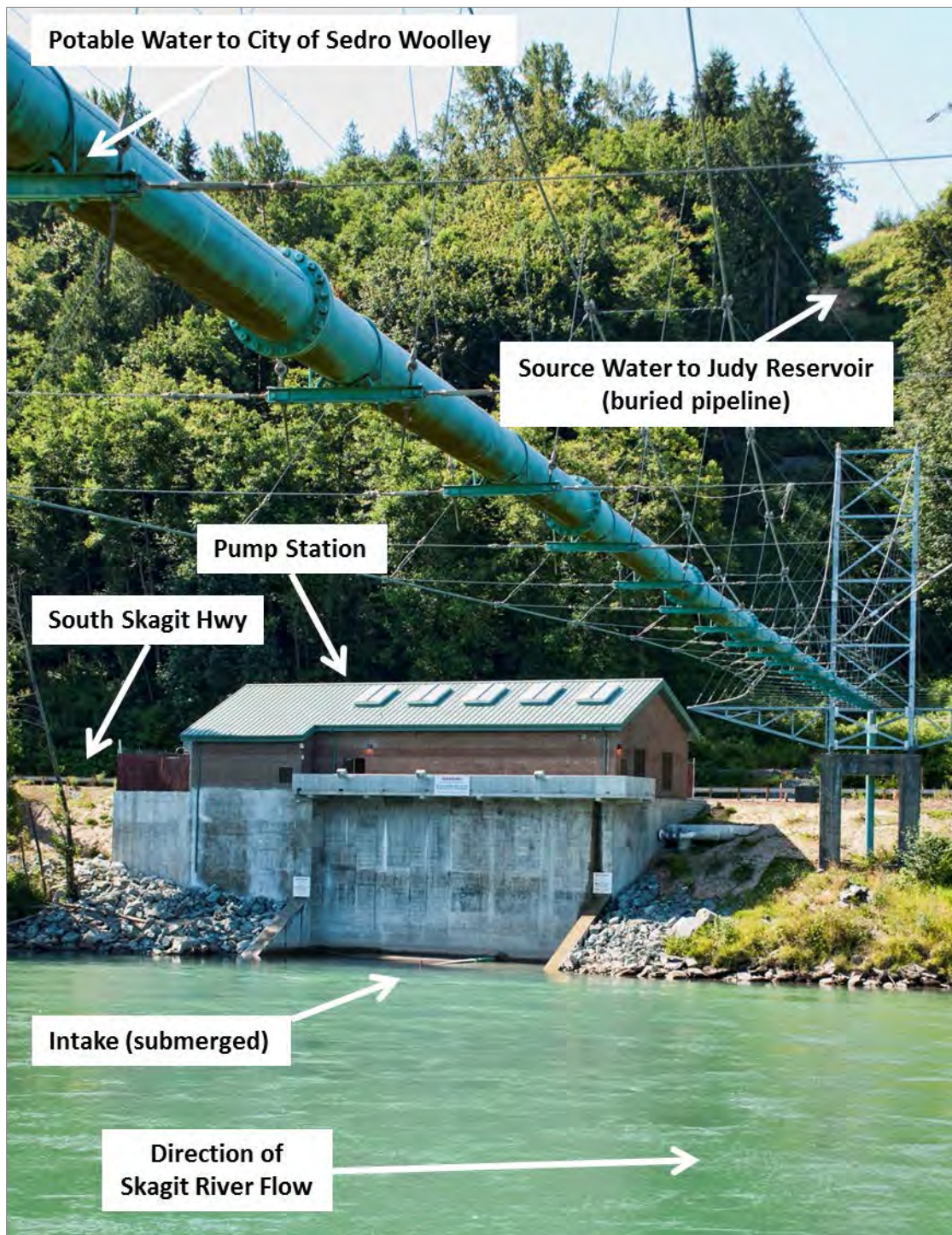
Figure 2-8. Skagit River Diversion Pump Station (SRD)
