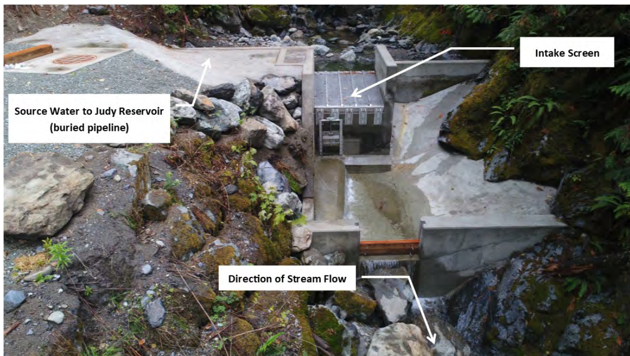
Figure 2-10. Mundt Creek Diversion
