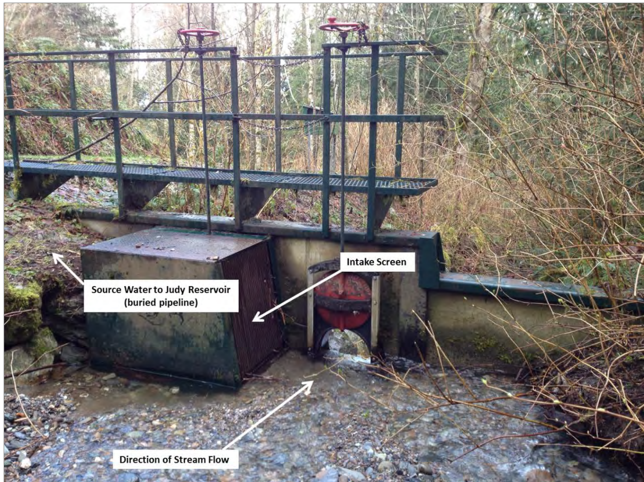
Figure 2-12. Salmon Creek Diversion
