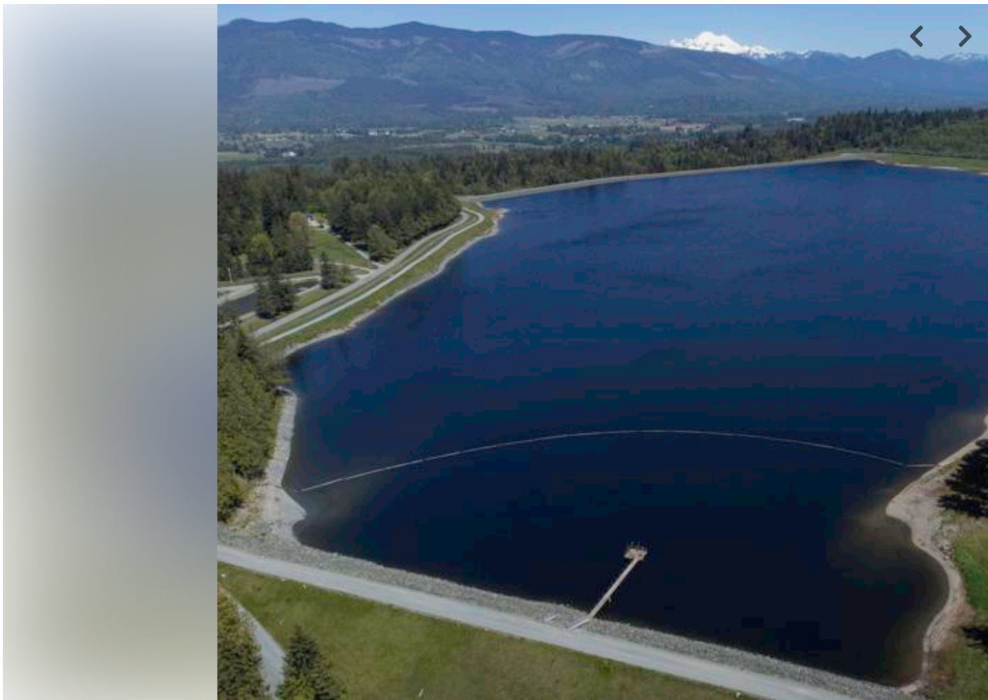
Judy Reservoir is pictured Thursday east of Clear Lake. When full, the lake is 60 feet deep and holds 1.5 billion gallons of water. Photo by Oliver Hamlin / Skagit Valley Herald
