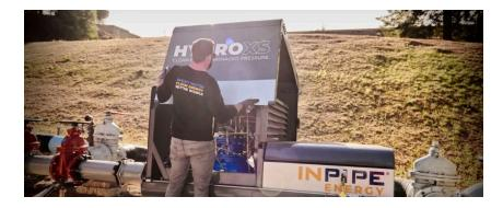
Skagit Public Utility District installed a power-producing pressure reduction valve to curb electric demand and carbon footprint.
