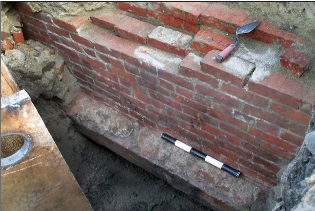
Figure B-6. Example of a historic building foundation.
